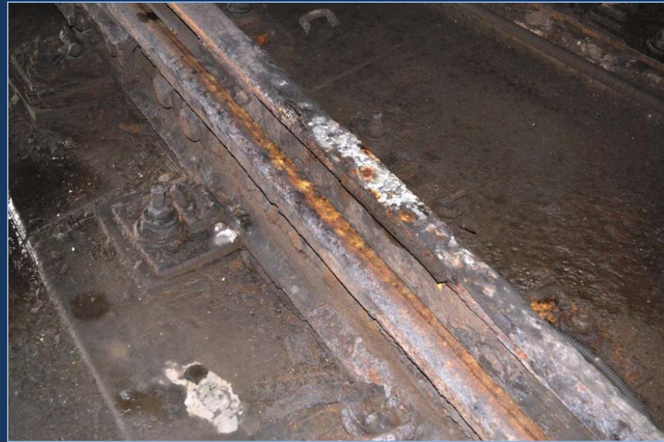
Corroded Running Rail
